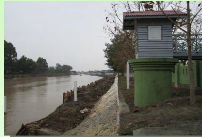
Discharge monitoring station
