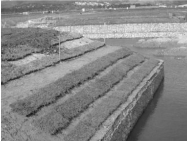
Fig. 7 Sod planting
