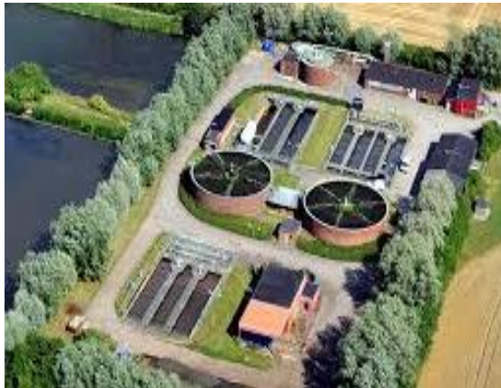
Improved sewage treatment in WWTP
