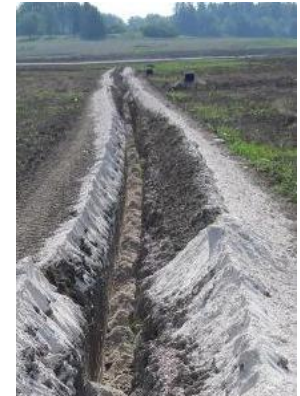
Lime-refill in sub-surface drainage
