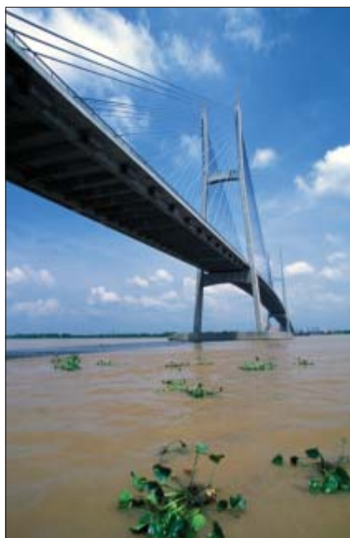
There are still very few bridges across the Mekong
