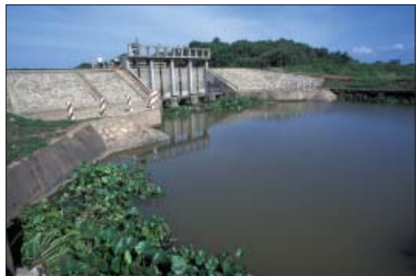
Dykes and other infrastructure protect delta farm land from salt water intrusion
