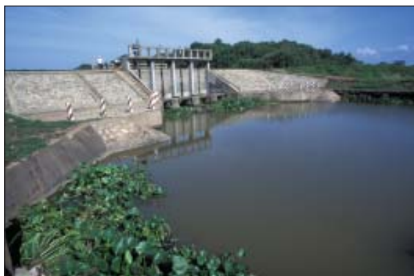
Barriers to stop sea water intrusion may prevent fish moving between the river and sea
