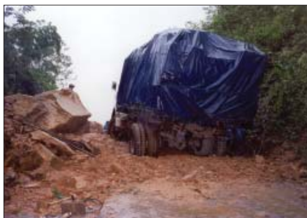
Lack of transportation infrastructure in the LMB impedes economic development
