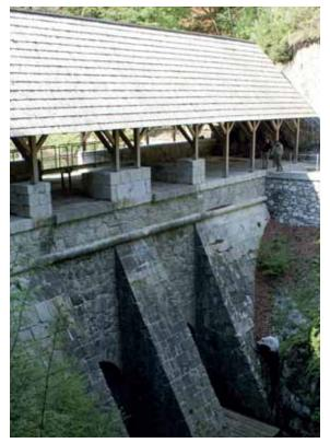
Photo B1-3: Energy demand: small hydropower station built during Napoleonic wars as dam for flushing timber and recently refurbished as small hydropower station. Kanomeljske klavže dam near Idrija, Slovenia.legame.
