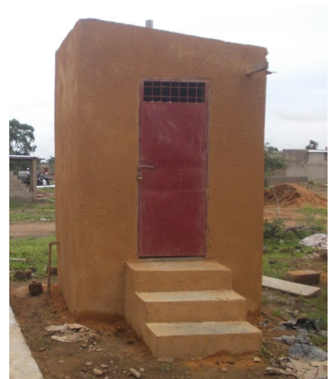
Ecosan Latrines © Koassanga Association
